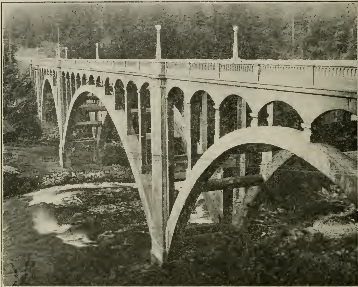
State Highway Bridge over the Sacramento River at Dunsmuir, showing use of California cement and crushed rock in a reinforced concrete structure.
